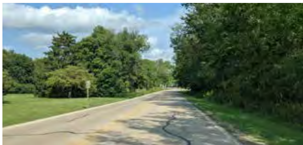
Existing conditions on Fire Lane 12
